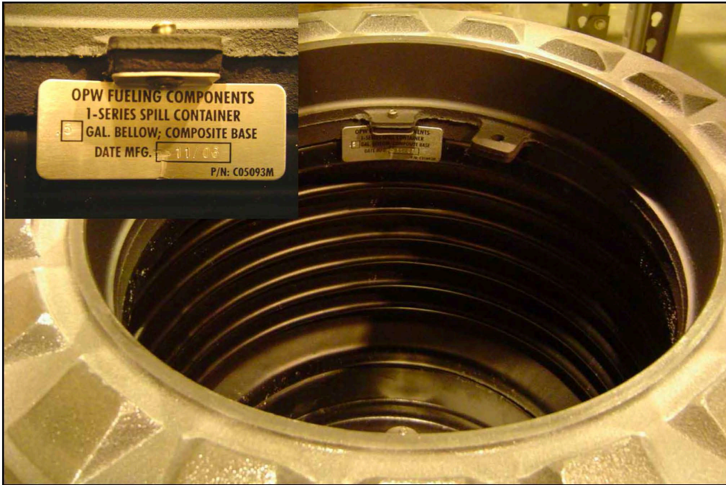
Figure 1-1 Direct Bury Spill Container OPW 1-Series (GAS/E85)
