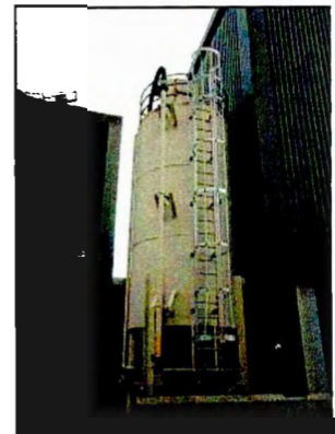
Fig. 2: The sand silo is located along the FBI building western edge.
