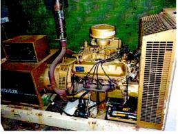
5.j <u>Camp Creek Radio Tower Emergency Generator Engine (new)</u>. The Camp Creek Radio Tower is powered by this engine when power from the solar array and battery system is not available. Equipment details are provided below:
