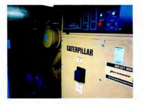
5.d <u>Swift #1 Dam Caterpillar Emergency Generator Engine</u>. This unit serves as an emergency power source for the fish sorting collector (FSC) for Swift Dam. Equipment details are provided below:
