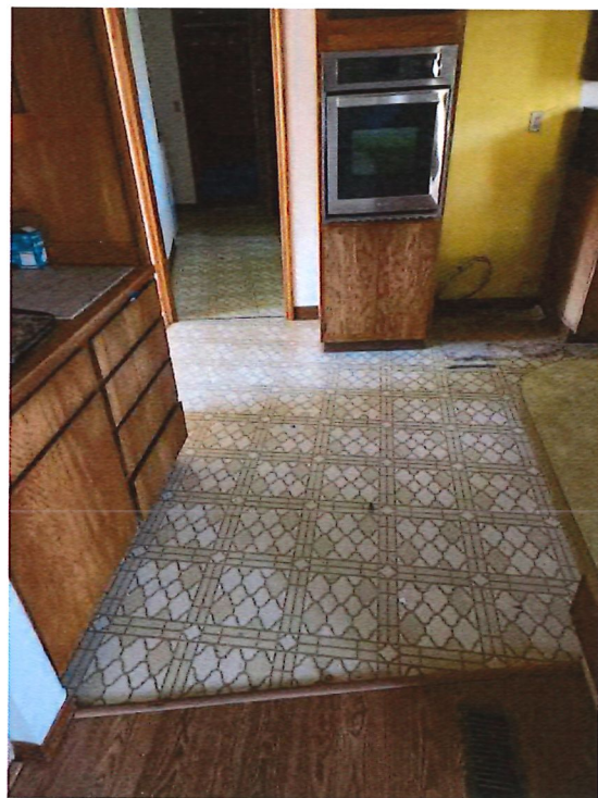
ASBESTOS FLOORING & MASTIC / KITCHEN - UT 18% CHRYSOTILE +/- 200 SQ/FT
