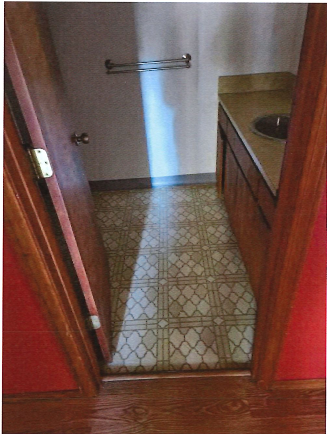
ASBESTOS FLOORING & MASTIC / KITCHEN - UT 18% CHRYSOTILE +/- 200 SQ/FT
