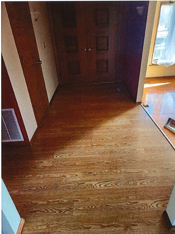
ASBESTOS FLOORING & MASTIC - ENTRANCE / UNDER WOOD - CHECK HALL & DINING ROOM 18% CHRYSOTILE +/- 200 SQ/FT
