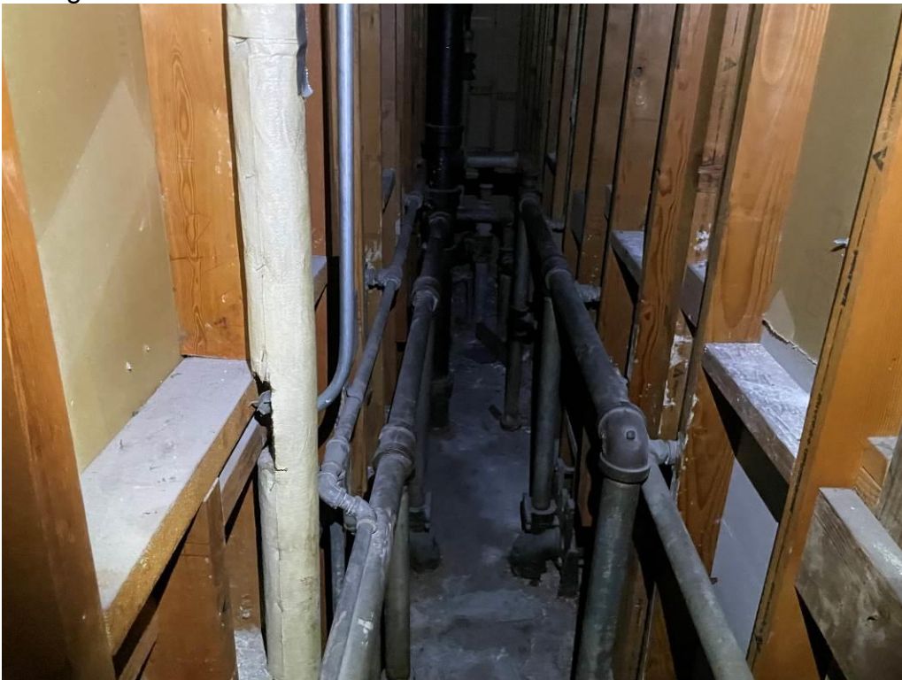
Photo 8: Mechanical chase closet located between the restrooms. The previously identified ACM pipe fitting insulation has been abated.
