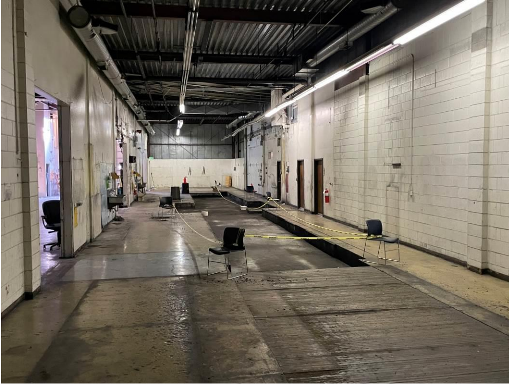
Photo 9: Press Room facing east. The SVF on the floor is asbestos containing.
