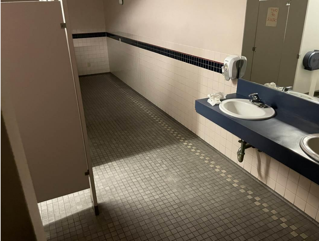
Photo 11: Assumed asbestos containing ceramic floor and wall tile mastic located in the restrooms.
