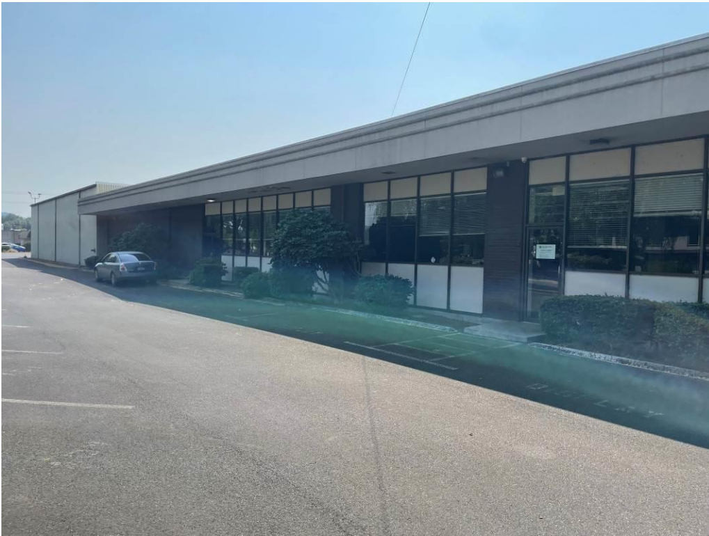
Photo 2: Exterior of the building facing southeast. The white window infill panels are cement asbestos board. The GWB soffit is also asbestos containing.
