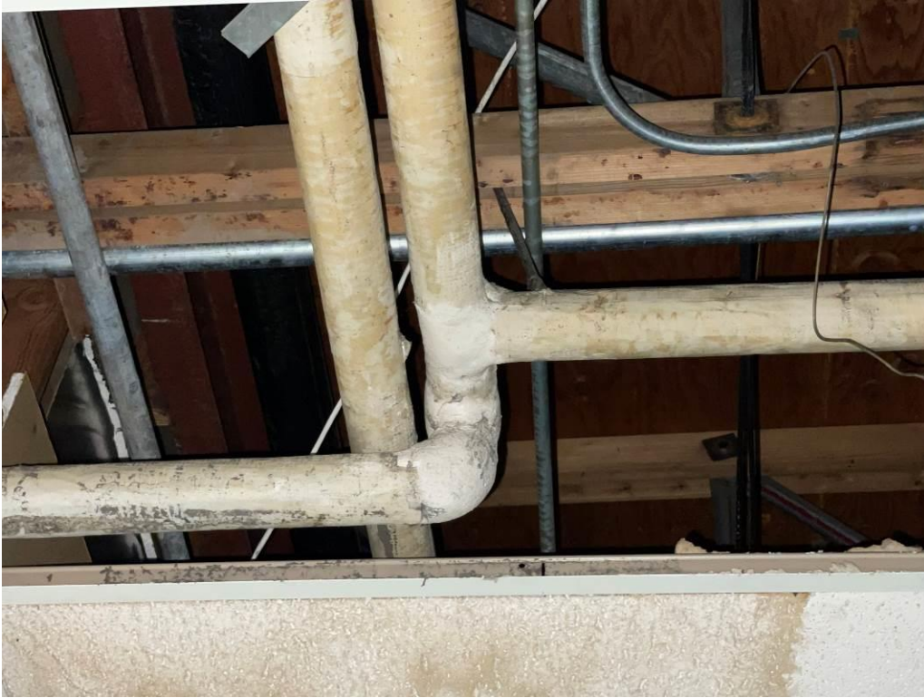
Photo 7: Asbestos containing mudded pipe fittings observed above the drop ceiling in the Mailroom.
