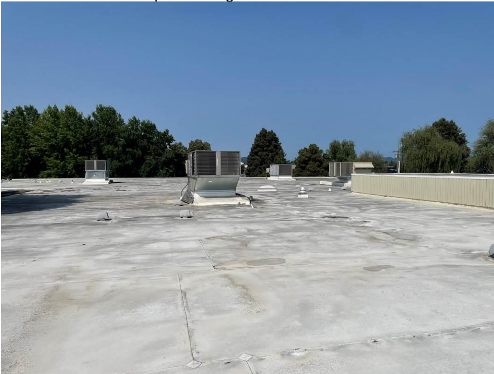
Photo 4: Roof of the building facing west. The roof is assumed ACM as it was unclear if existing layers of roofing are present underneath the white sealed membrane.
