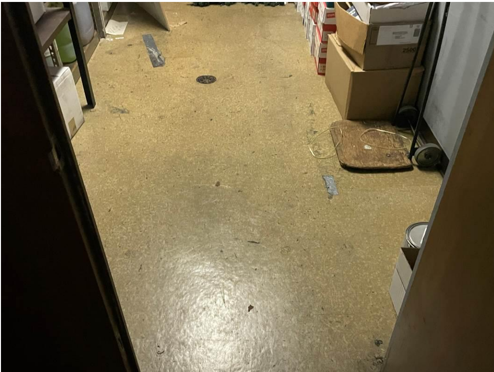
Photo 12: Asbestos containing SVF in the Plate Making storage room.
