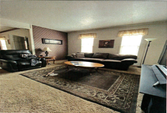
Living room with 2 layers of carpet on vinyl sheeting floor, and sheetrock walls and ceiling with brocade texture.
