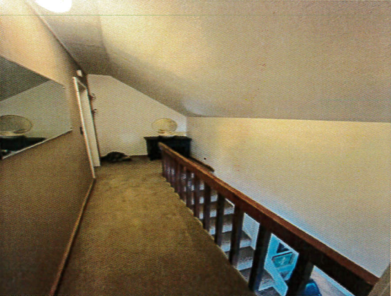
Upstairs hallway with carpet on original hardwood, one wood panel wall and three sheetrock walls and ceiling with brocade texture.
