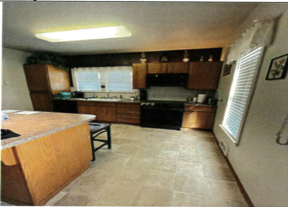
Kitchen with 2 layers of vinyl sheeting floor, and sheetrock walls and ceiling with brocade texture.
