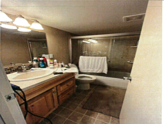
Bathroom with 2 layers of vinyl sheeting floor, and sheetrock walls and ceiling with brocade texture.
