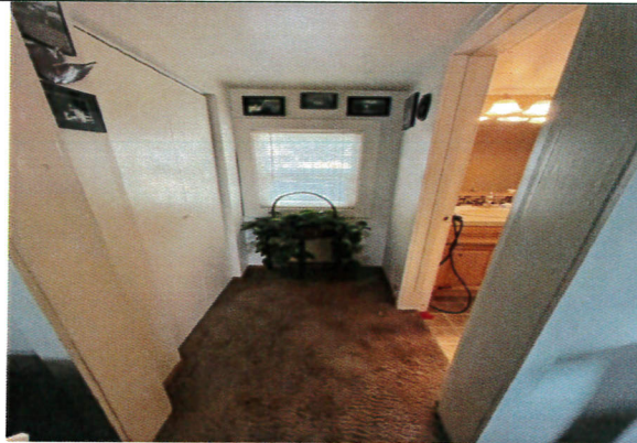
Hallway with carpet floor, and sheetrock walls and ceiling with brocade texture.
