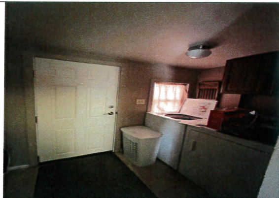
Utility with 2 layers of vinyl sheeting floor, and sheetrock walls and ceiling with brocade texture.
