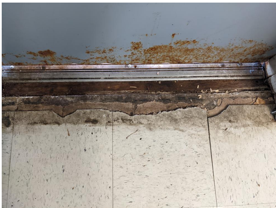
Photo 4 HA-3: 8"x8" tan vinyl floor tile (2# Chrysotile) and black mastic (4% Chrysotile).
