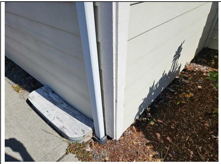
3. Exterior: painted plank siding and wood trim.
