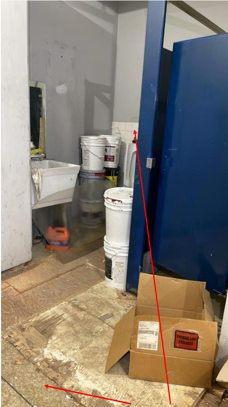
Mezzanine restroom (back) ACM vinyl and pipe fitting insulation (hard).
