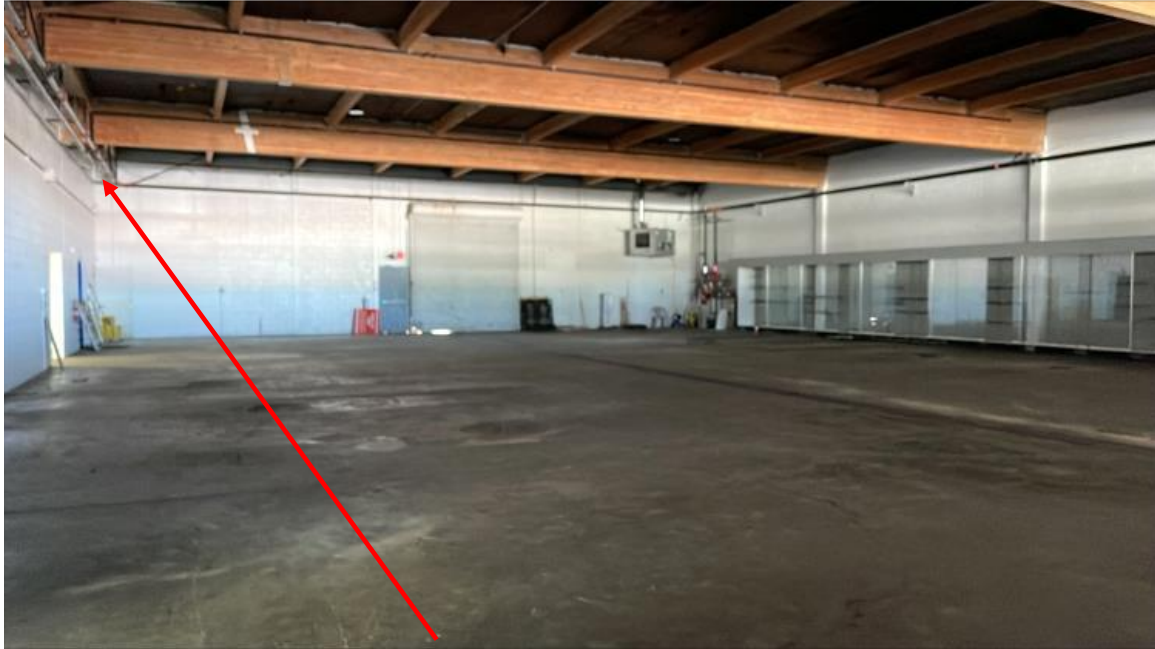
Shop area ACM pipe fitting insulation (hard)
