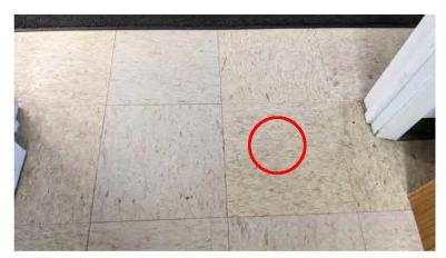
Photo 2 — HA-4: Off-white, brown-mottled vinyl floor tiles (non-ACM) with tan mastic (non-ACM) and residual black mastic (3% chrysotile), located in the western offices and as patching throughout the project area
