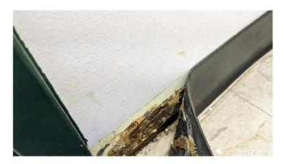
Photo 4 – White on yellow paint on gypsum wallboard and wood associated with walls in the east restroom of Building PC0602 (Sample: PC0602-PC-4, 360 ppm)
