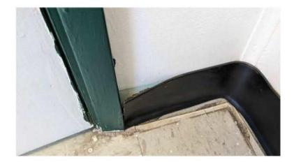
Photo 3 – White on light green paint on gypsum wallboard and wood associated with walls throughout Building PC0602 (Sample: PC0602-PC-3, 340 ppm).
