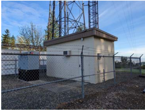
Southeast exterior elevation viewing northwest
