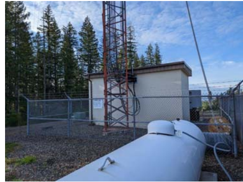
Northwest exterior elevation viewing southeast
