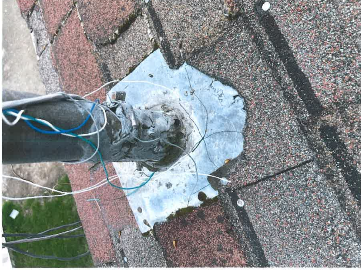
Photo shows black penetration mastic (gray oxidized outer surface) located and adhered to a pipe, roof flashing made of lead, and 3-tab roofing. This material contains 5% chrysotile asbestos.
