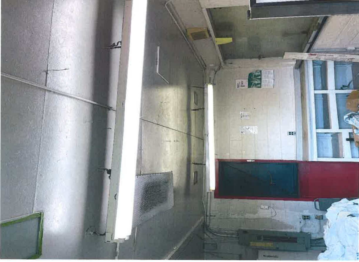
Photo shows four (4) 8 feet long fluorescent light tubes and two fixtures. These tubes and ballast will need to be recycled or disposed of as universal waste. There are a total of eight (8), eight-foot tubes and 8 to 12 light ballast from 4 fixtures. The ballast will need to be checked to determine if they are PCB-containing or not for proper disposal. Check label to see if the ballast indicates Non-PCB Containing.
