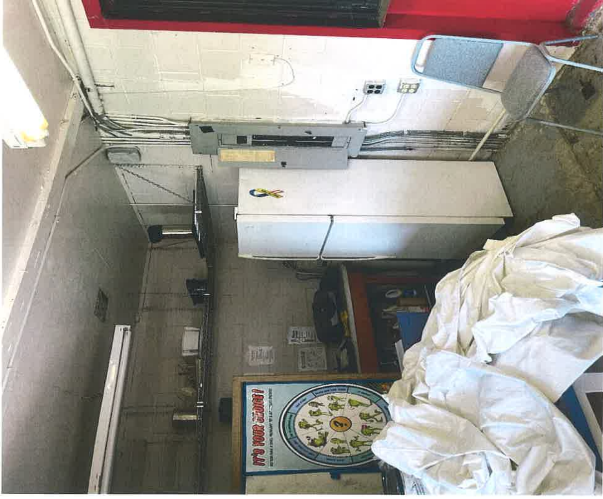
Photo shows the same black asbestos-containing floor mastic from a former floor tile application, where it ends just past the chair. Note: Much of this black mastic has a paint like coating on top of it. This material contains 5-6% chrysotile asbestos.
