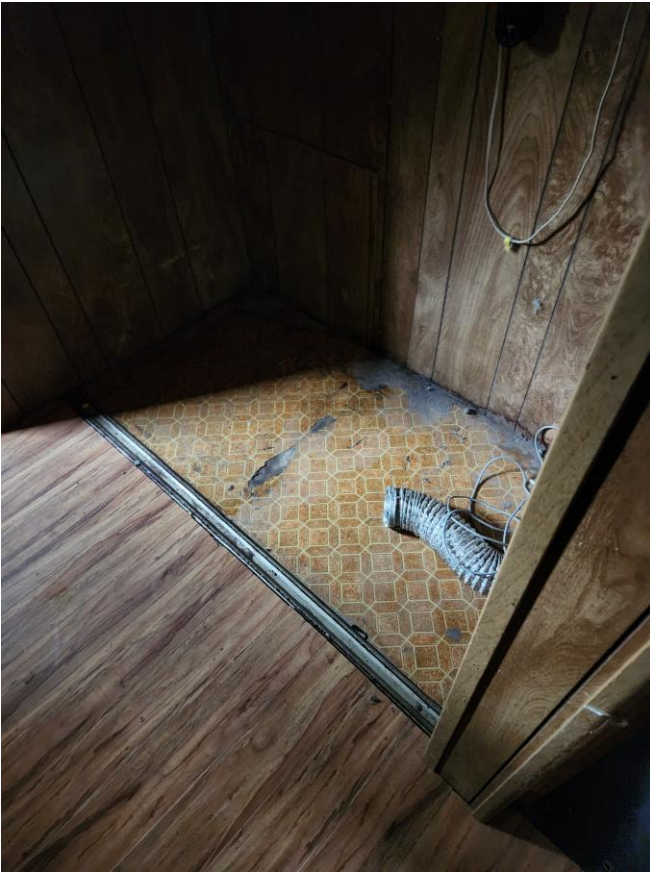
F-3 & 4 ASBESTOS FLOORING – KITCHEN AREA - +/- 250 sq/ft (UNDER LAMINANT)
