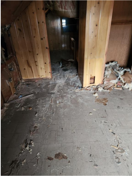
F-3 - ASBESTOS FLOORING – 9X9 – UPSTAIRS AREA - +/- 400 sq/ft
