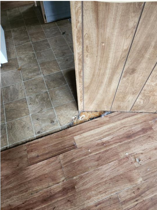
F-3 & 4 ASBESTOS FLOORING – KITCHEN AREA - +/- 250 sq/ft (UNDER LAMINANT)
