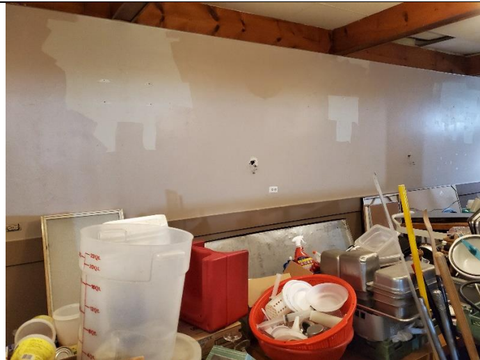
PHOTO 003 – Samples 119 and 120 Asbestos-Containing Joint Compound on Gypsum Wallboard
