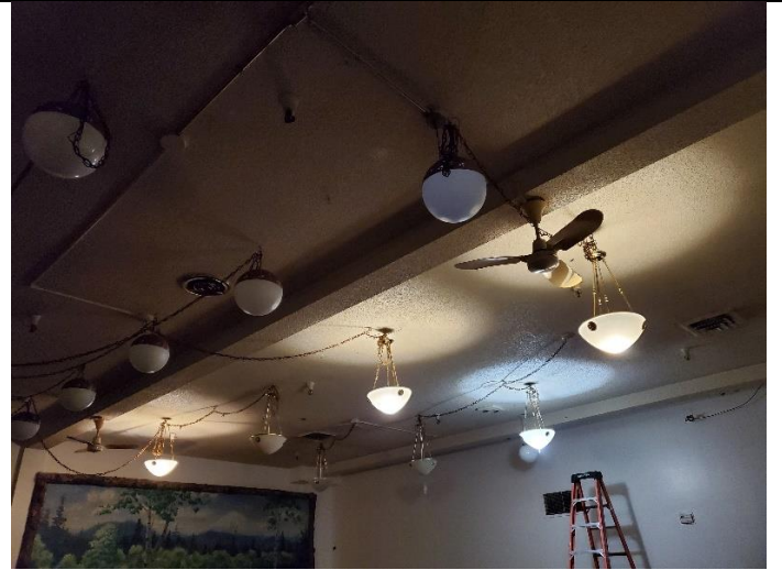
PHOTO 002 – Samples 108, 109, and 110 Asbestos-Containing Ceiling Texture in Banquet Room
