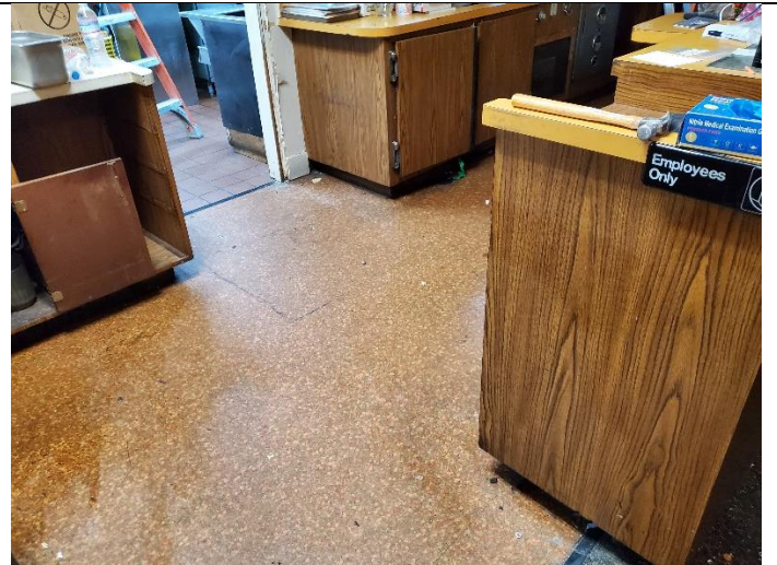
PHOTO 004 – Sample 121 Asbestos-Containing Sheet Vinyl Flooring in Serving Area
