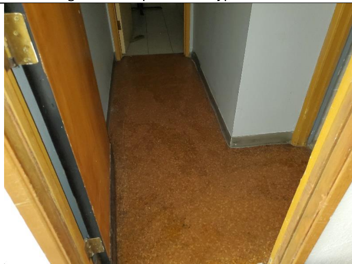
PHOTO 005 – Sample 123 Asbestos-Containing Sheet Vinyl Flooring in Rest Room Hallway
