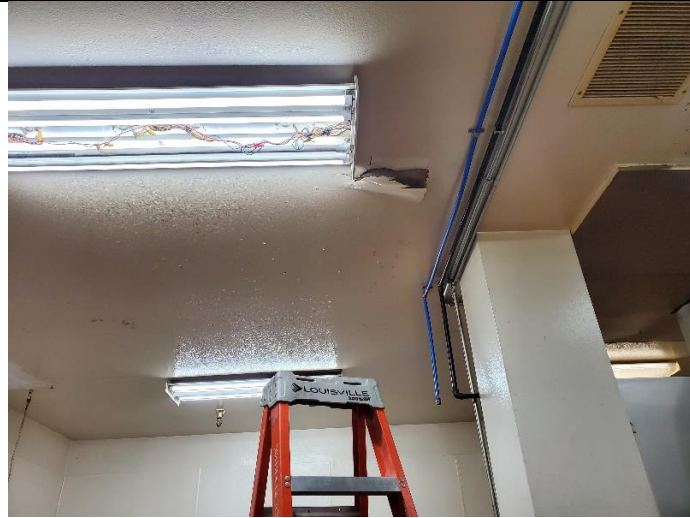
PHOTO 001 – Samples 106 and 107 Asbestos-Containing Texture Paint on Kitchen Ceiling
