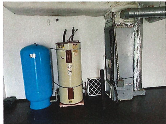
Photo #2 View of water pressure tank, water heater, and furnace located in garage of 1201 parcel large house
